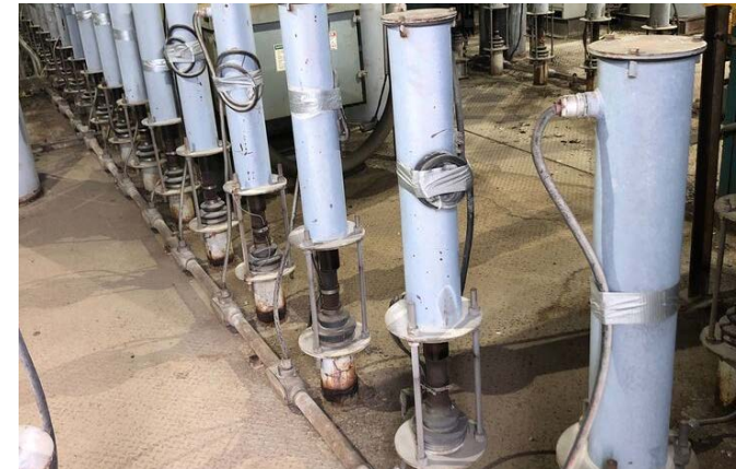
Collector Plate Tumble Hammer Rappers
